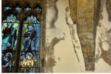
As is common in historic buildings, salts form on the walls in some areas indicating moisture movement in the fabric. Monitoring humidity over time will show whether this is transferring to the internal environment to cause people to feel cold, or enabling algal growth.
