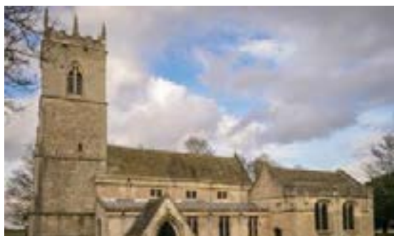
St Katherine’s Church (Exterior)
