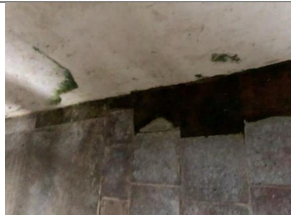
Patches of damp can be a sign that drainage around a building is not working correctly. Check corresponding drains, guttering and downpipes
